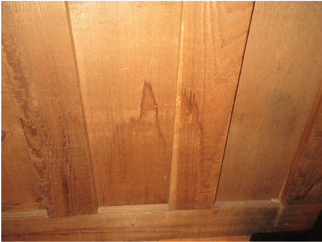
16-Man Cave Date Taken: 5/22/2025 Taken By: Michael Wallen Water damage to paneling.
