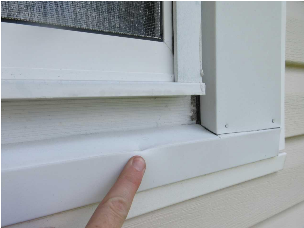
119-S Rear Elevation Date Taken: 6/27/2025 Taken By: Michael Wallen Hail damage to window wrap.
