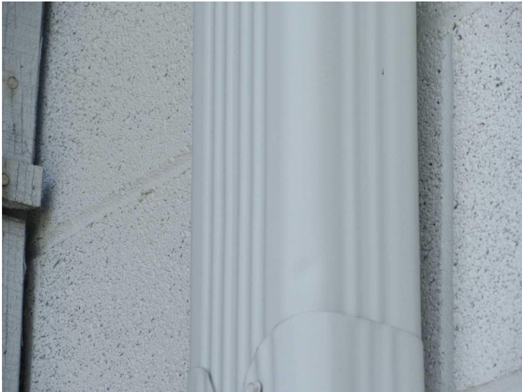
5-W Rear Elevation Date Taken: 6/27/2025 Taken By: Michael Wallen Hail damage to downspout.
