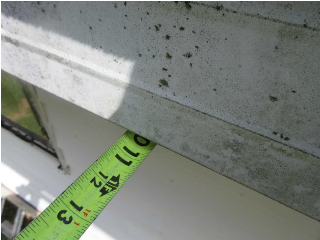
89-Soffit Date Taken: 6/27/2025 Taken By: Michael Wallen 10" soffit.
