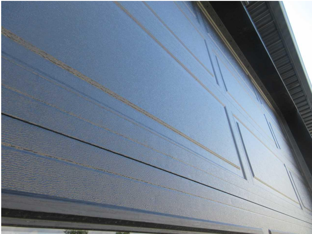
155-W Front Elevation Date Taken: 6/27/2025 Taken By: Michael Wallen Hail damage to overhead door.
