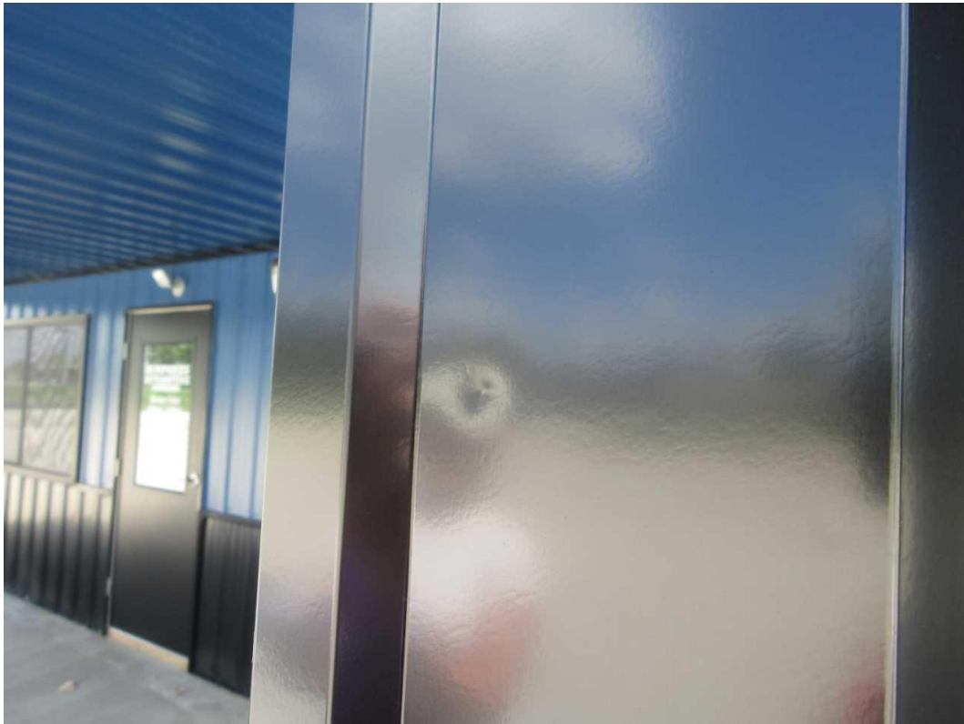
151-W Front Elevation Date Taken: 6/27/2025 Taken By: Michael Wallen Hail damage to post wraps.
