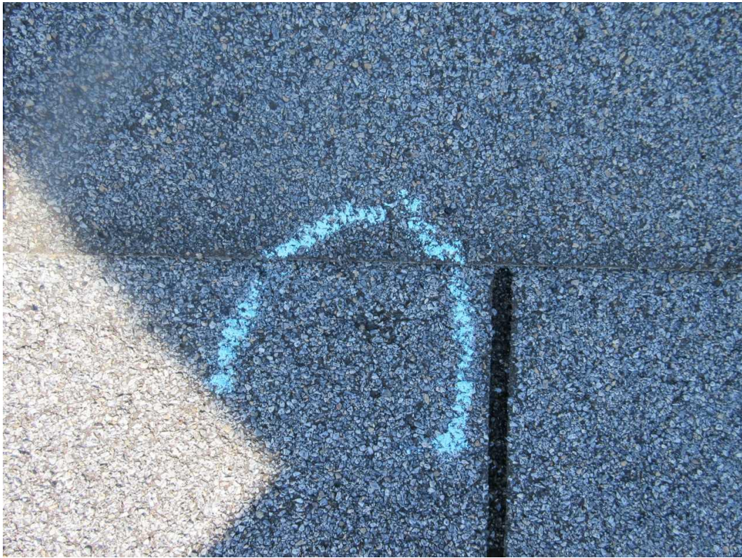
16-E Front Slope Date Taken: 6/27/2025 Taken By: Michael Wallen Close up of hail damage inside the test square.
