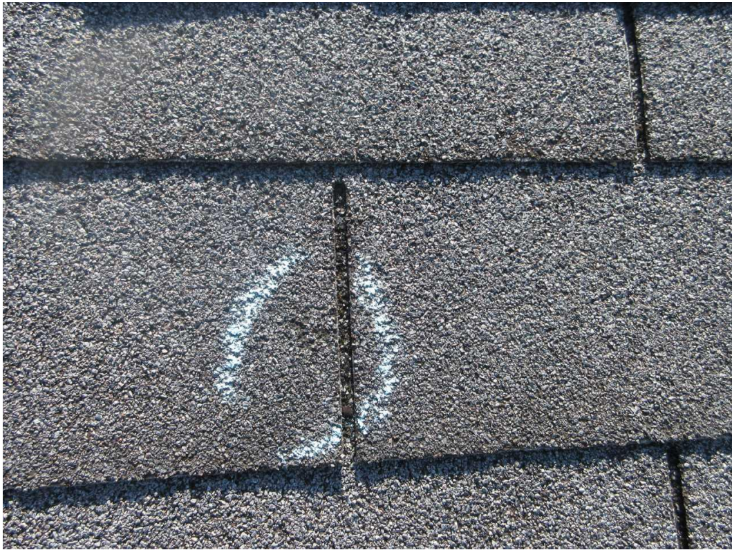
18-W Back Slope Date Taken: 6/27/2025 Taken By: Michael Wallen Close up of hail damage inside the test square.
