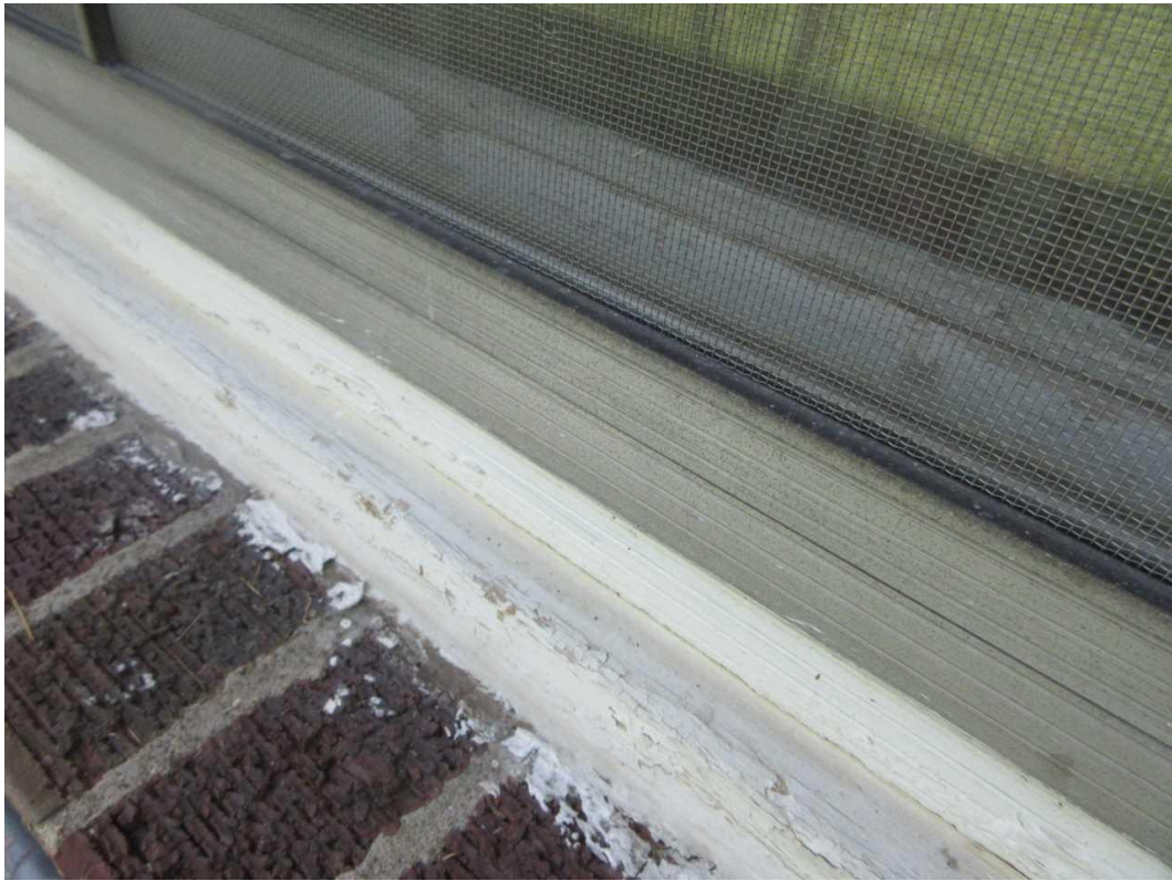
46-W Rear Elevation Date Taken: 6/27/2025 Taken By: Michael Wallen Hail damage to paint on the wood windows.
