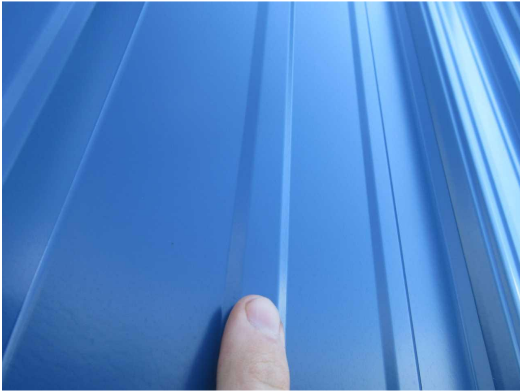
152-W Front Elevation Date Taken: 6/27/2025 Taken By: Michael Wallen Hail damage to metal siding.
