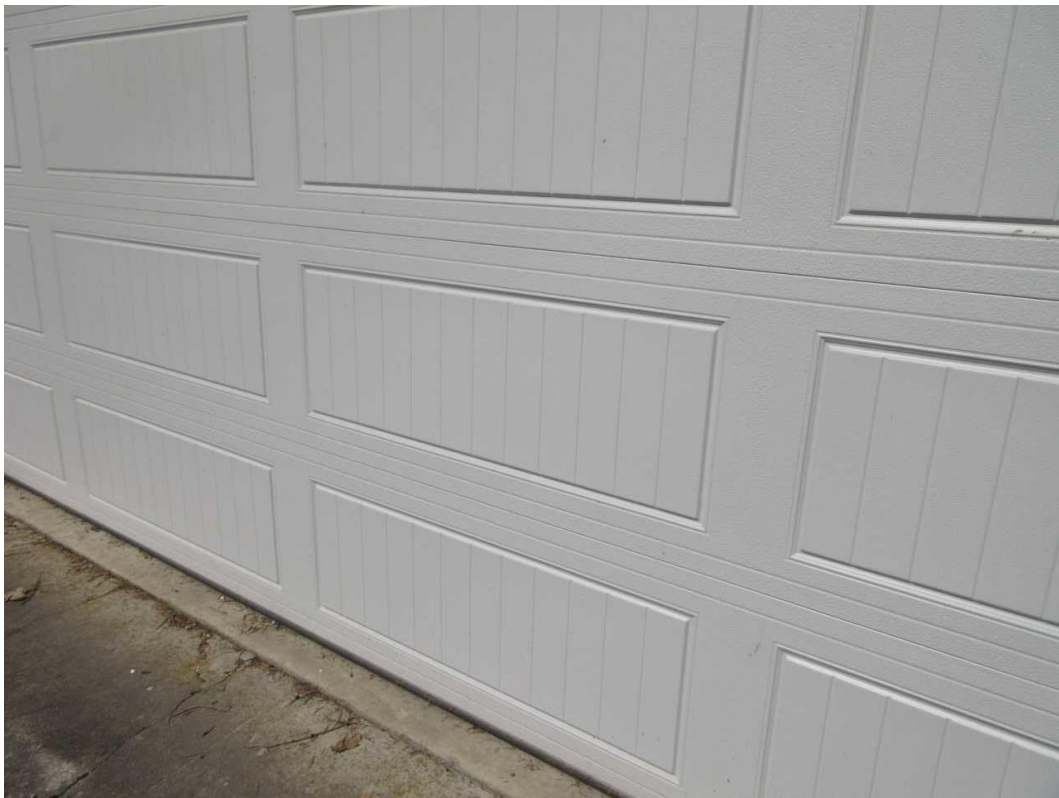
81-E Front Elevation Date Taken: 6/27/2025 Taken By: Michael Wallen No storm damage to overhead door from the claimed date of loss.
