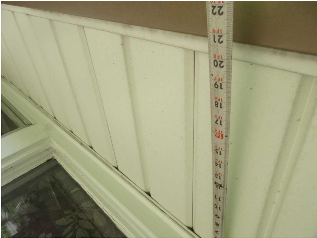
62-Soffit Date Taken: 6/27/2025 Taken By: Michael Wallen 1'9" soffit.
