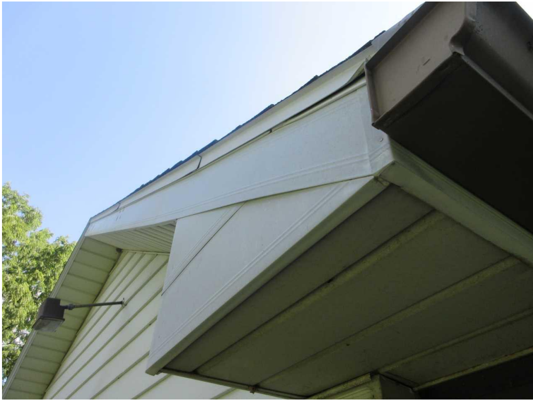
38-W Rear Elevation Date Taken: 6/27/2025 Taken By: Michael Wallen Hail damage to fascia.
