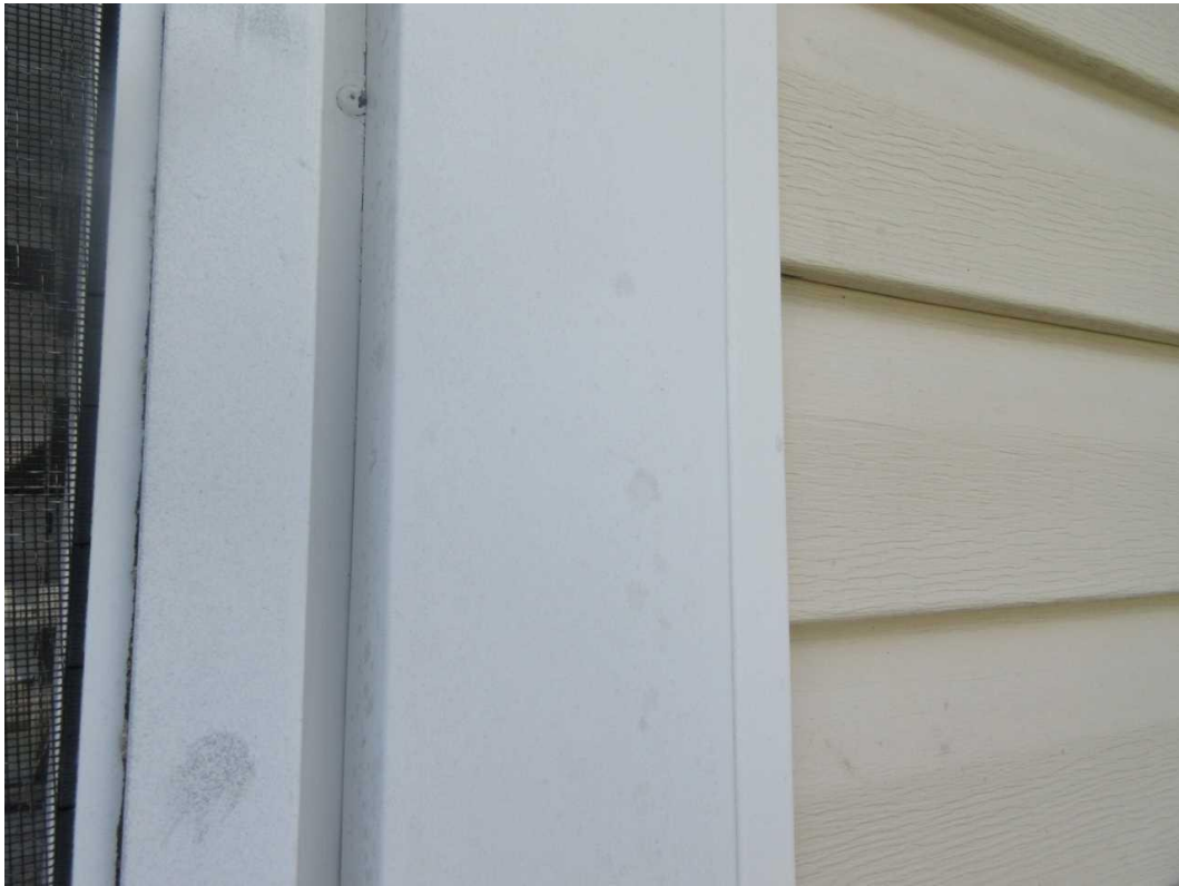
103-W Right Elevation Date Taken: 6/27/2025 Taken By: Michael Wallen Hail damage to window wrap.
