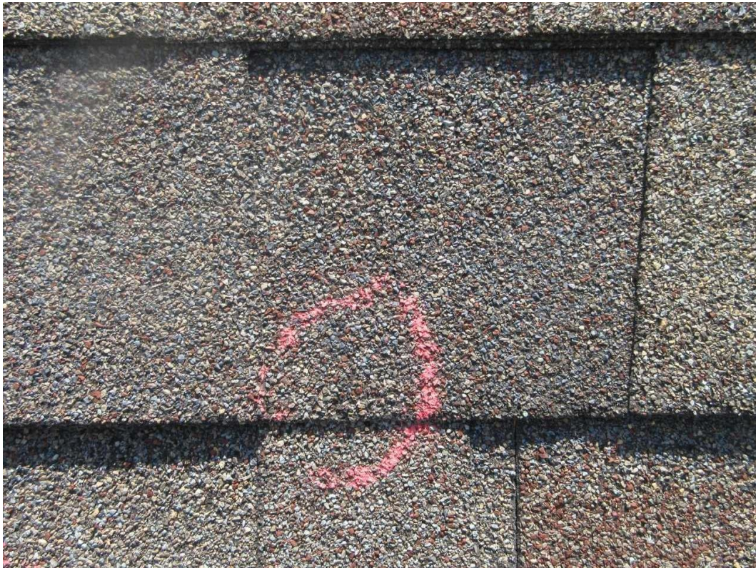
71-W Back Slope Date Taken: 6/27/2025 Taken By: Michael Wallen Close up of hail damage inside the test square.
