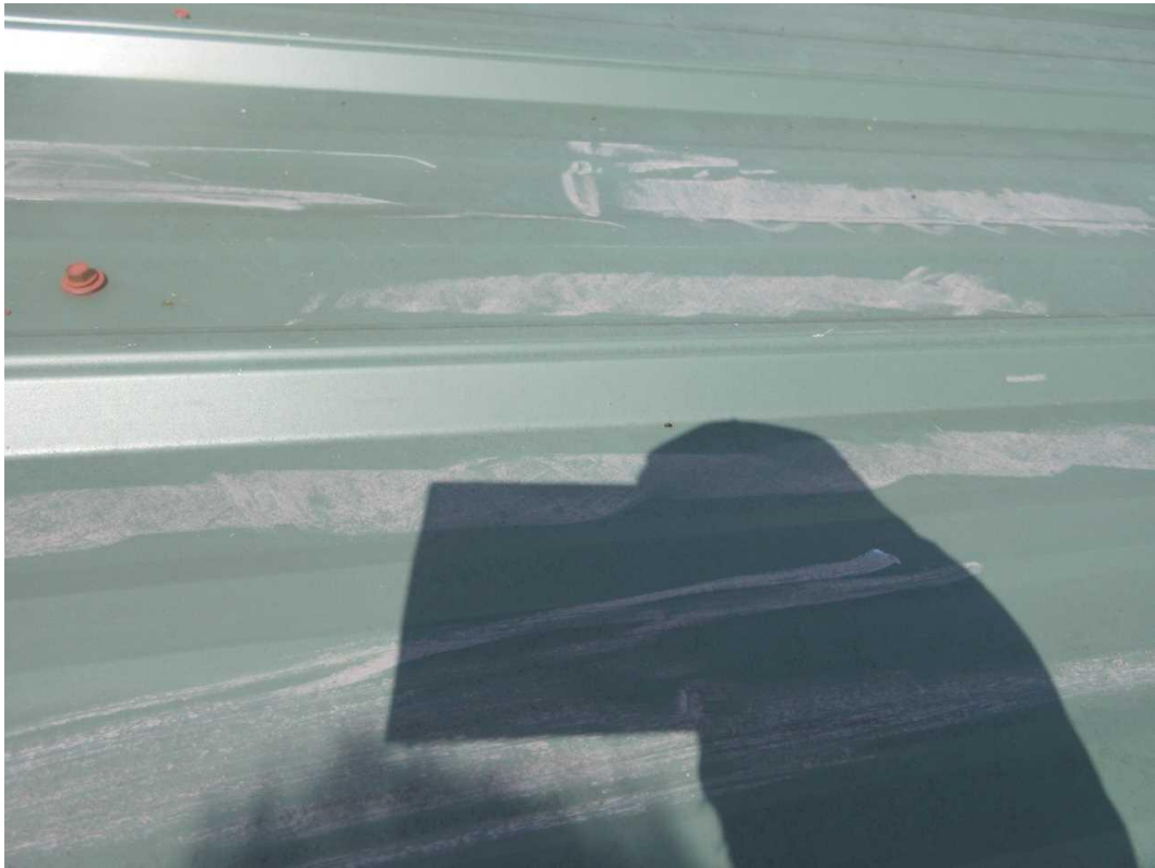
133-Ribbed Metal Roof Date Taken: 6/27/2025 Taken By: Michael Wallen Hail damaged.
