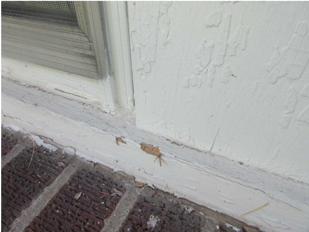
45-W Rear Elevation Date Taken: 6/27/2025 Taken By: Michael Wallen Hail damage to paint on the wood windows.
