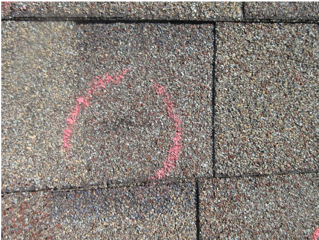
78-S Left Slope Date Taken: 6/27/2025 Taken By: Michael Wallen Close up of hail damage inside the test square.
