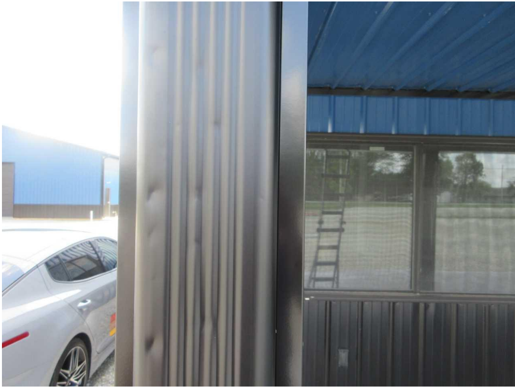
150-W Front Elevation Date Taken: 6/27/2025 Taken By: Michael Wallen Hail damage to downspout
