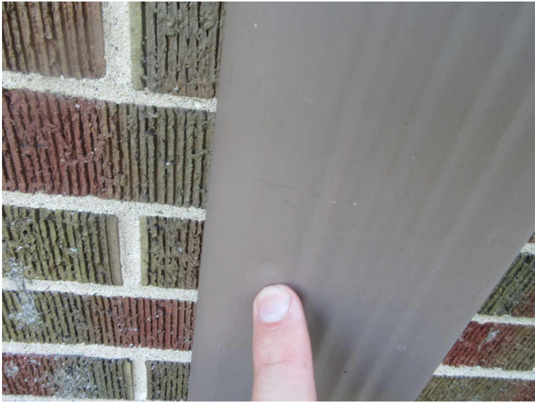
34-W Rear Elevation Date Taken: 6/27/2025 Taken By: Michael Wallen Hail damage to downspout.
