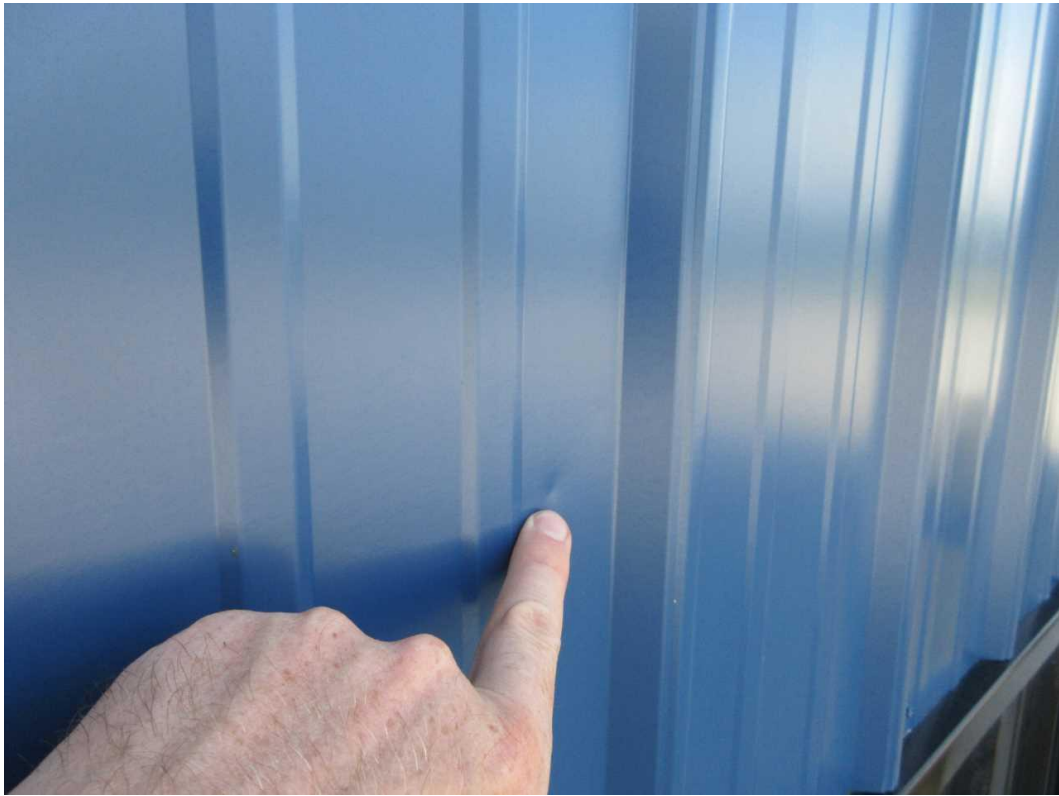
160-W Front Elevation Date Taken: 6/27/2025 Taken By: Michael Wallen Hail damage to metal siding.
