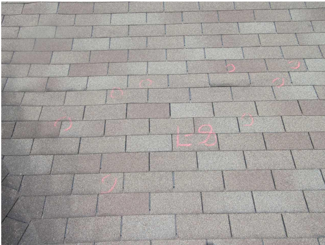
145-E Left Slope Date Taken: 6/27/2025 Taken By: Michael Wallen Overview of the test square.
