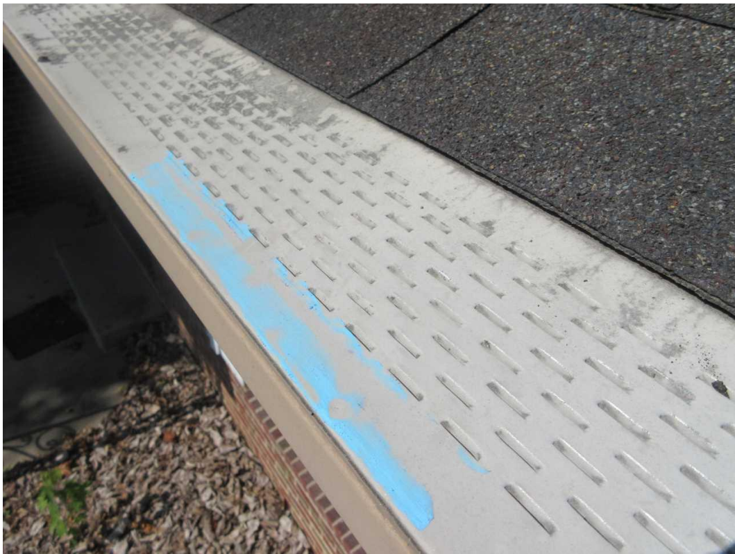
61-Gutters Date Taken: 6/27/2025 Taken By: Michael Wallen Hail damage to gutter guard.
