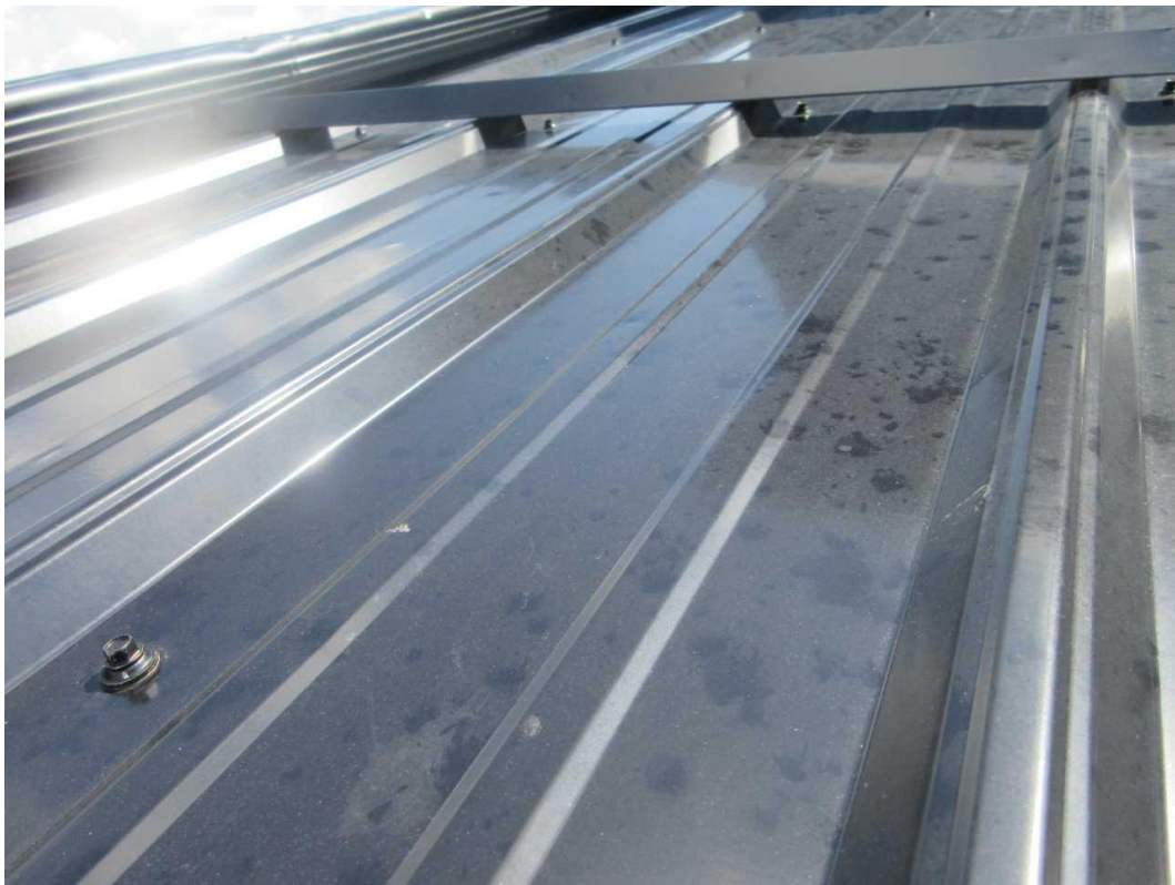
185-Roof Date Taken: 6/27/2025 Taken By: Michael Wallen Hail damage to ribbed metal roofing.
