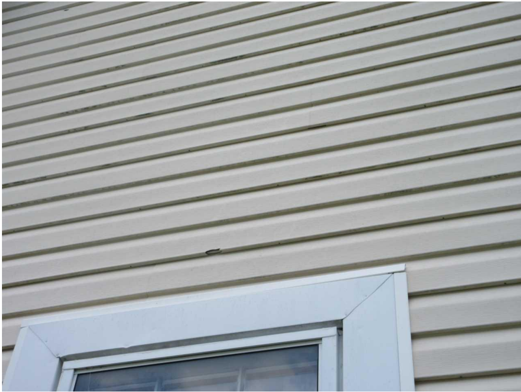
112-W Right Elevation Date Taken: 6/27/2025 Taken By: Michael Wallen Hail damage to vinyl siding.
