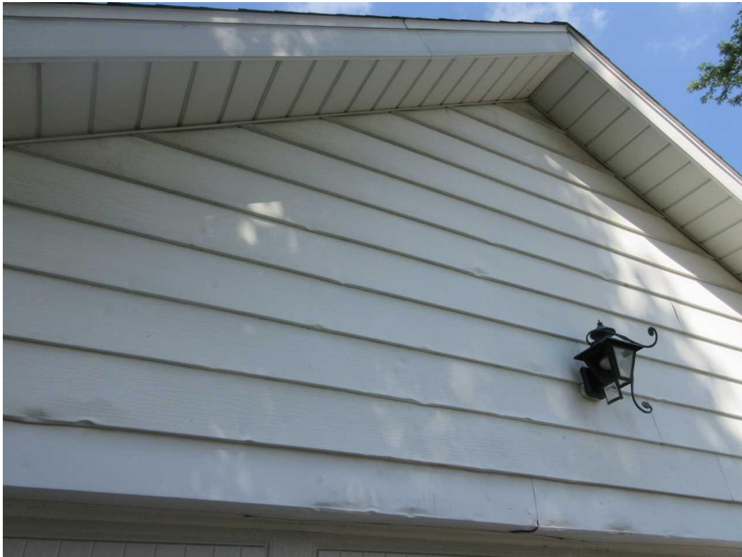
29-E Front Elevation Date Taken: 6/27/2025 Taken By: Michael Wallen Mechanical damage to aluminum siding.
