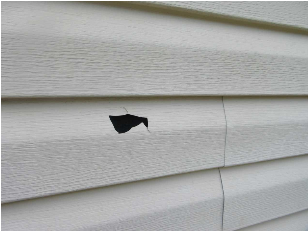
111-W Right Elevation Date Taken: 6/27/2025 Taken By: Michael Wallen Hail damage to vinyl siding.
