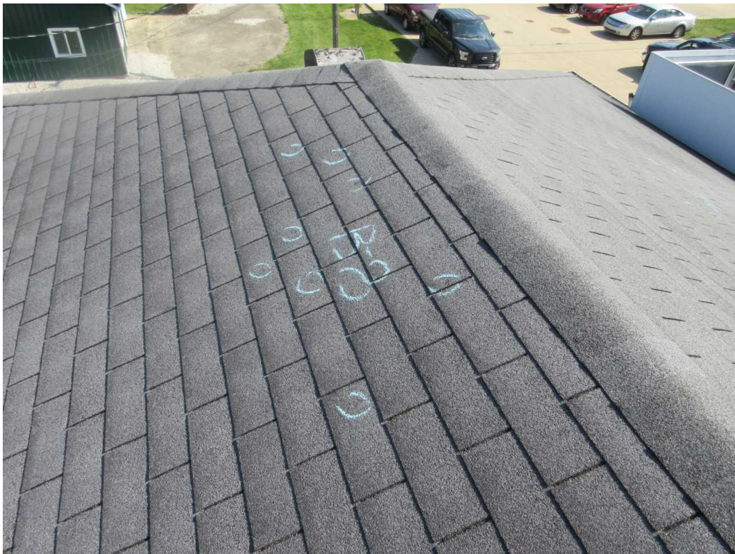
17-W Back Slope Date Taken: 6/27/2025 Taken By: Michael Wallen Overview of the test square.
