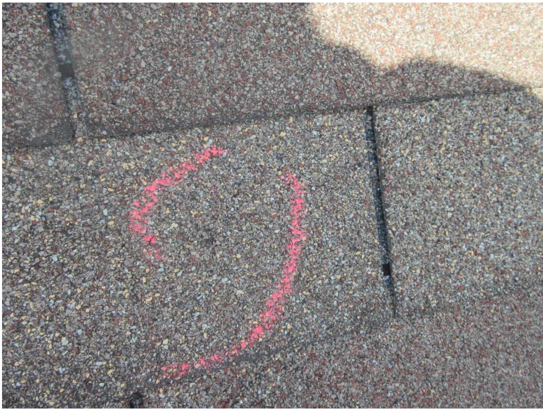
146-E Left Slope Date Taken: 6/27/2025 Taken By: Michael Wallen Close up of hail damage inside the test square.
