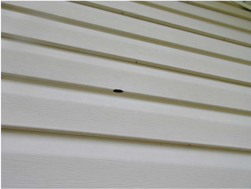
110-W Right Elevation Date Taken: 6/27/2025 Taken By: Michael Wallen Hail damage to vinyl siding.
