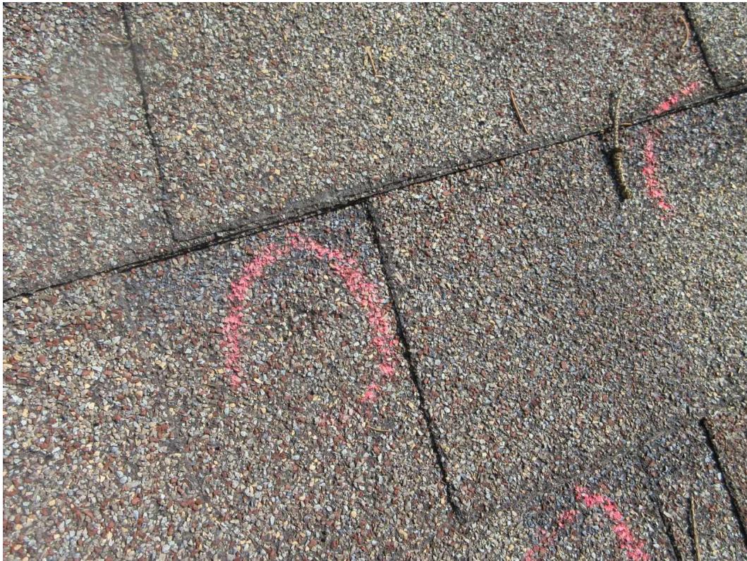
97-S Left Slope Date Taken: 6/27/2025 Taken By: Michael Wallen Close up of hail damage inside the test square.
