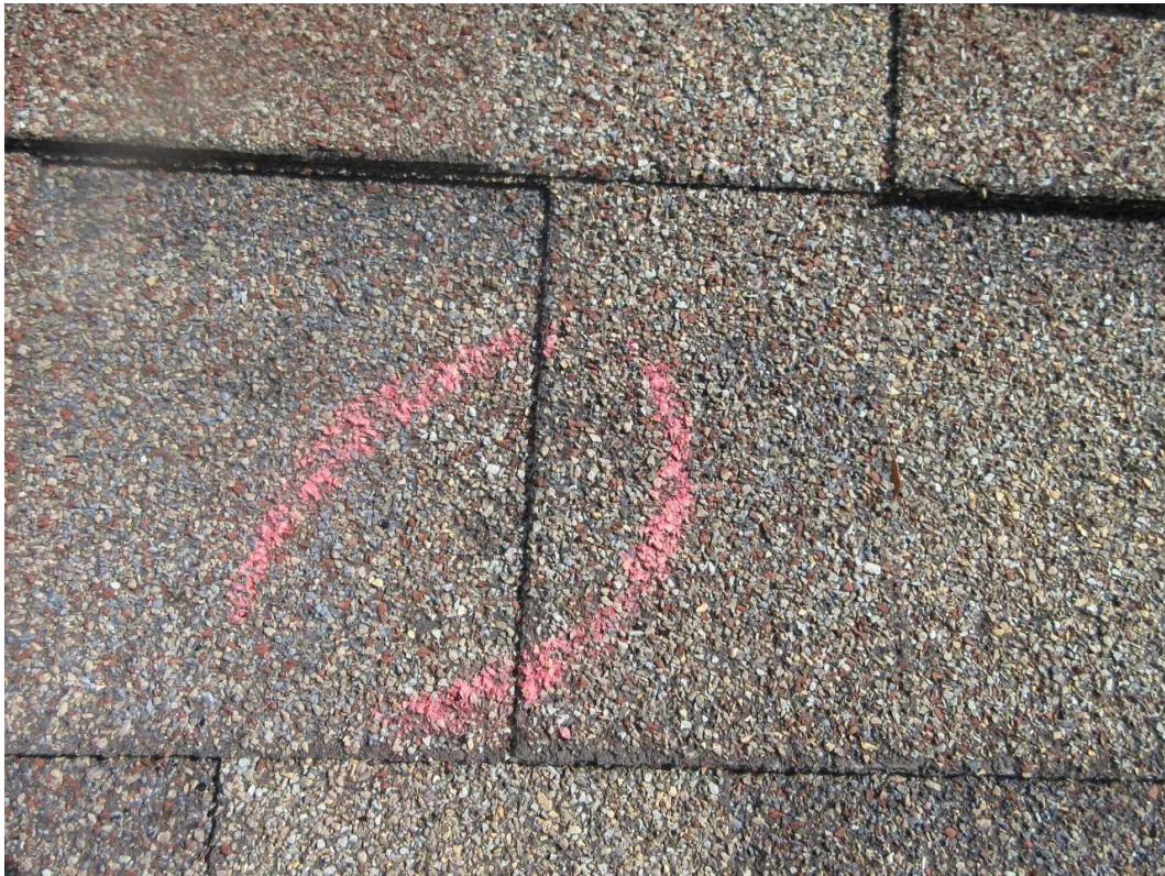
79-S Left Slope Date Taken: 6/27/2025 Taken By: Michael Wallen Close up of hail damage inside the test square.
