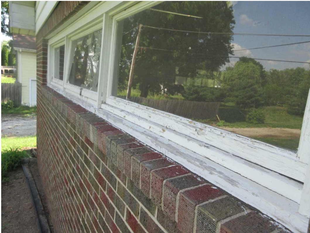
41-W Rear Elevation Date Taken: 6/27/2025 Taken By: Michael Wallen Hail damage to paint on the wood windows.
