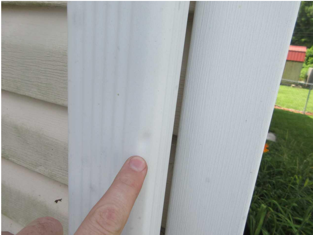
101-N Front Elevation Date Taken: 6/27/2025 Taken By: Michael Wallen Hail damage to downspout.
