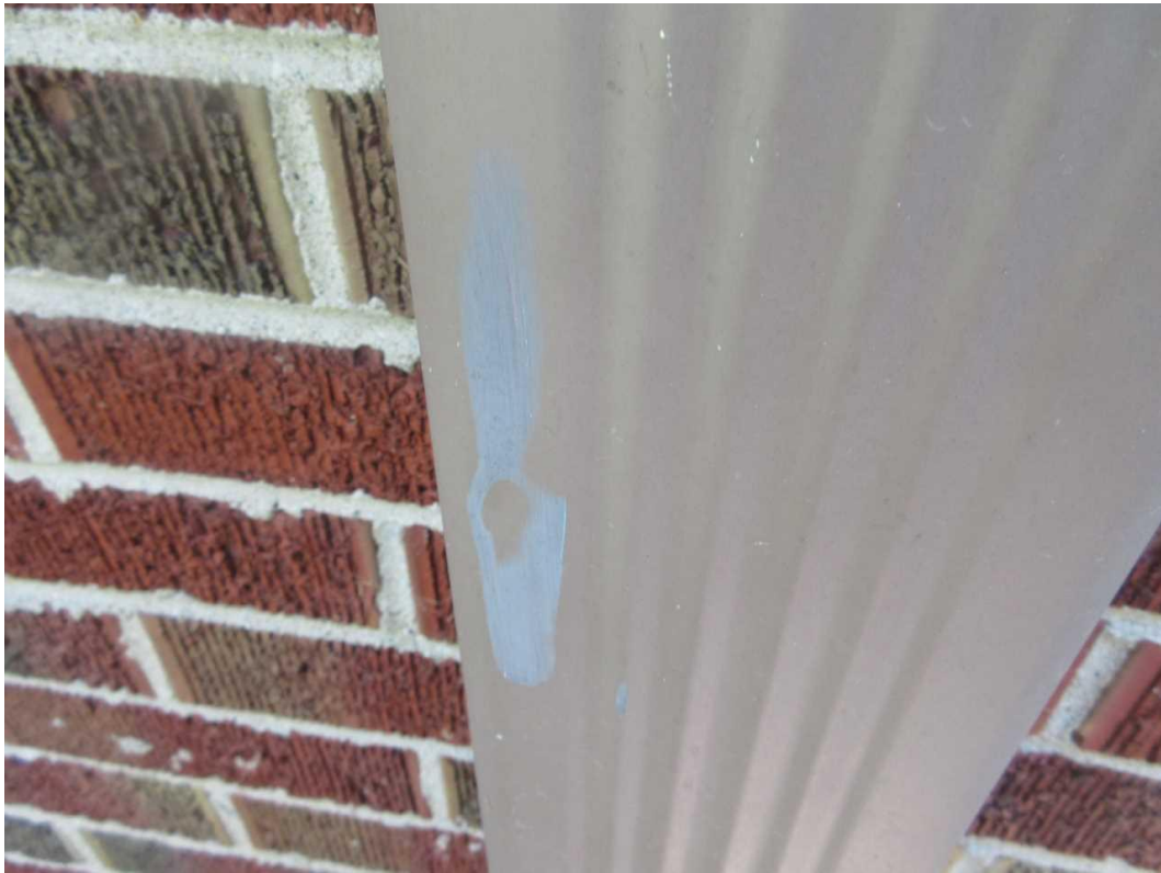
47-W Rear Elevation Date Taken: 6/27/2025 Taken By: Michael Wallen Hail damage to downspout.
