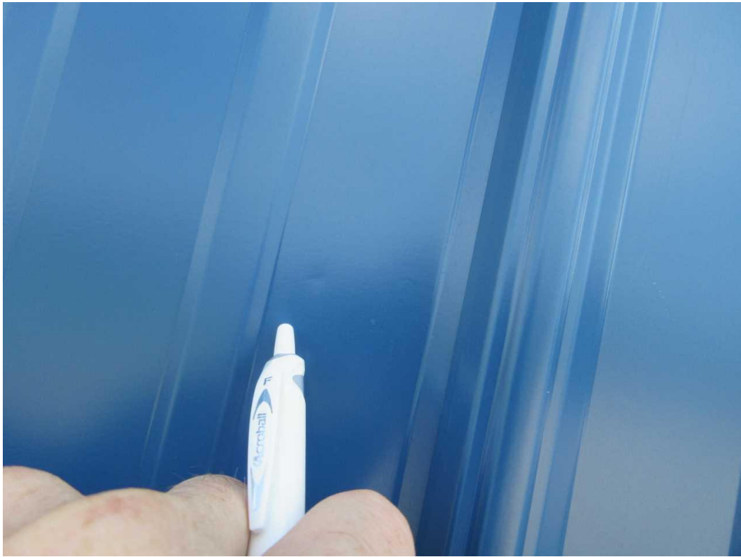
188-W Front Elevation Date Taken: 6/27/2025 Taken By: Michael Wallen Hail damage to metal siding.
