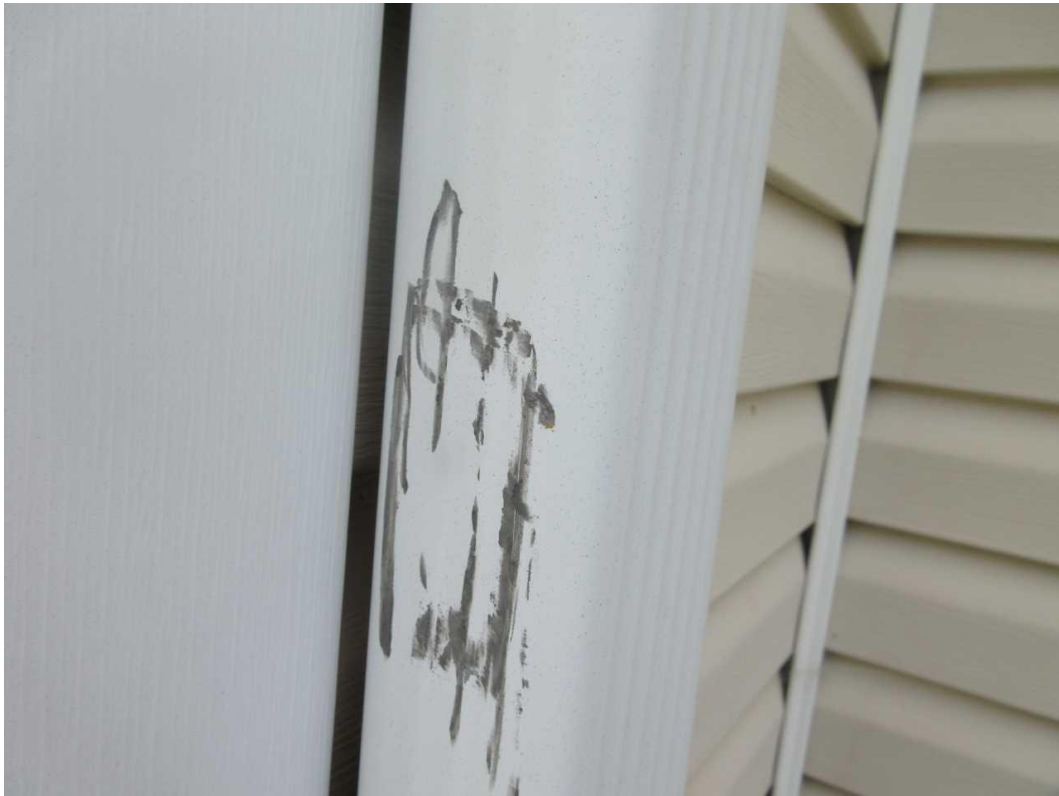
107-W Right Elevation Date Taken: 6/27/2025 Taken By: Michael Wallen Hail damage to downspout.
