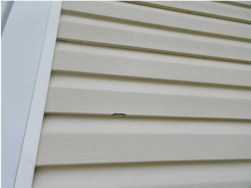
109-W Right Elevation Date Taken: 6/27/2025 Taken By: Michael Wallen Hail damage to vinyl siding.
