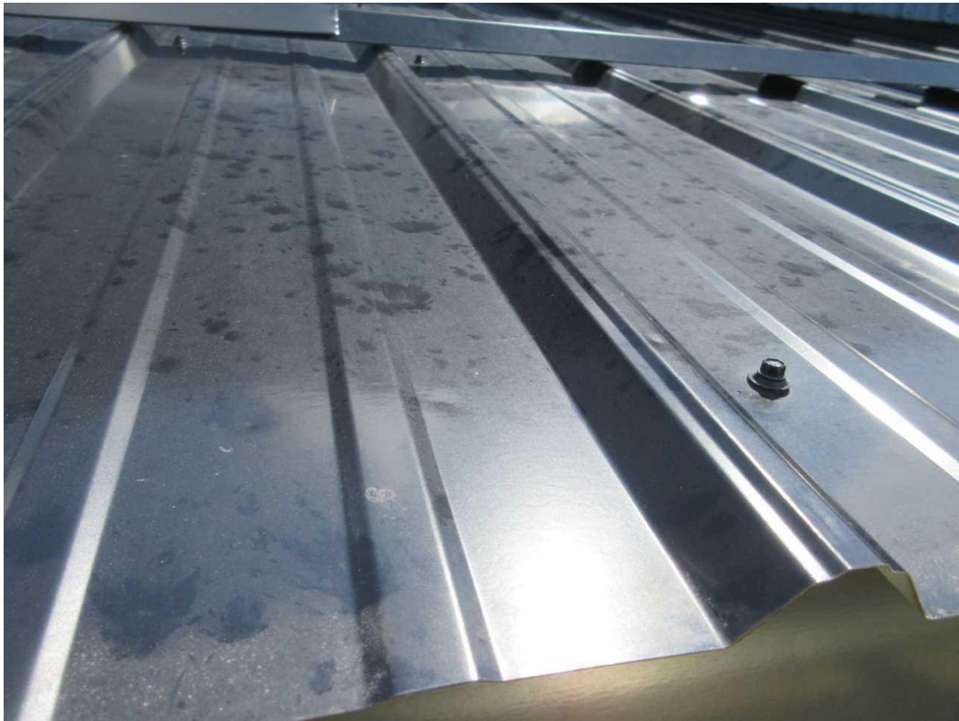
183-Roof Date Taken: 6/27/2025 Taken By: Michael Wallen Hail damage to ribbed metal roofing.
