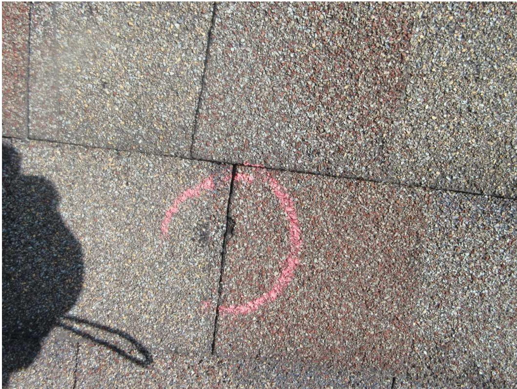
77-S Left Slope Date Taken: 6/27/2025 Taken By: Michael Wallen Close up of hail damage inside the test square.
