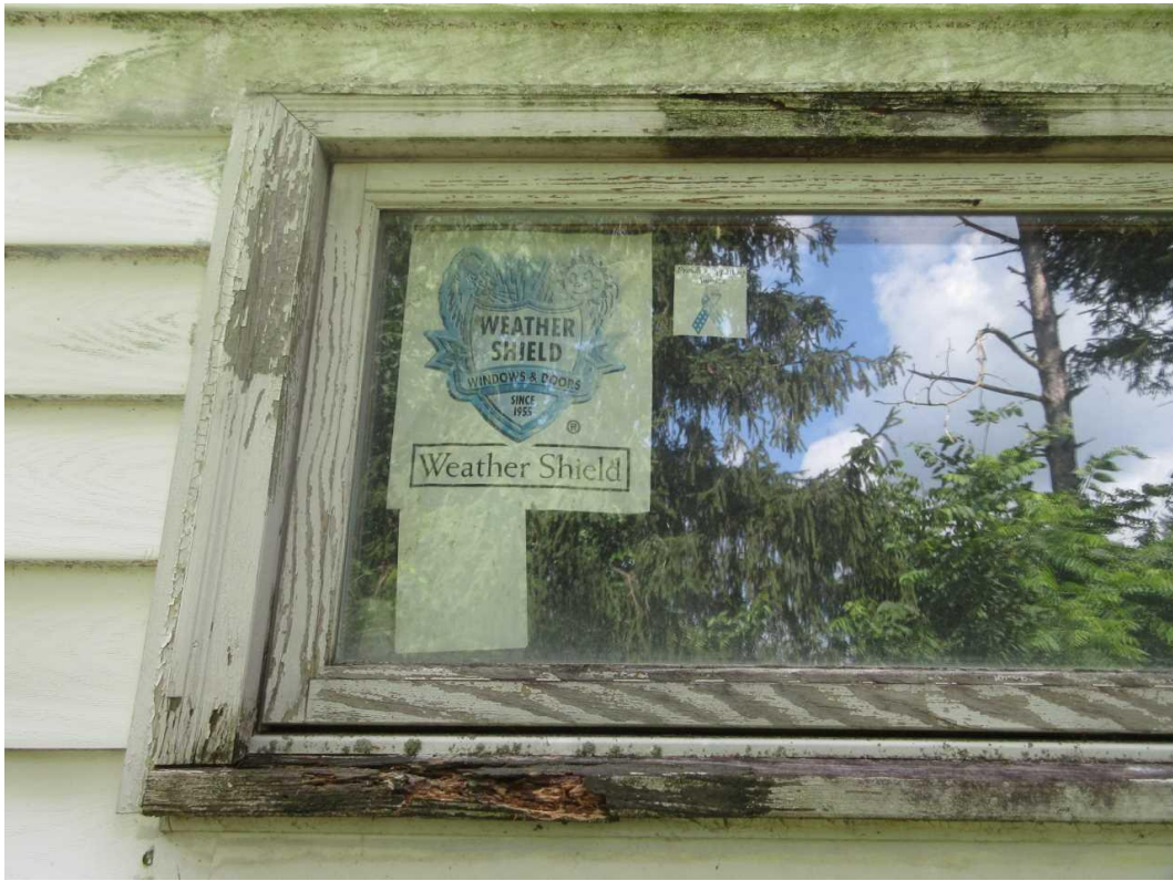
84-W Rear Elevation Date Taken: 6/27/2025 Taken By: Michael Wallen Pre-existing condition of window, not storm related.
