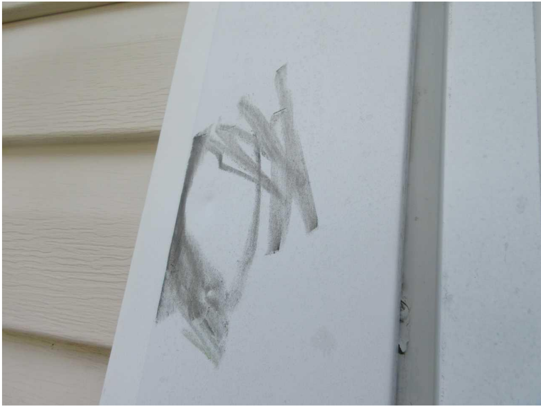
104-W Right Elevation Date Taken: 6/27/2025 Taken By: Michael Wallen Hail damage to window wrap.
