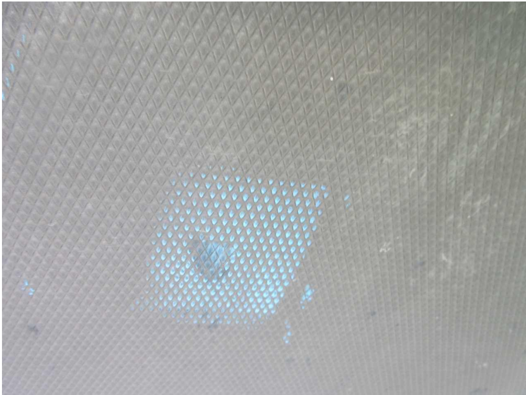
37-W Rear Elevation Date Taken: 6/27/2025 Taken By: Michael Wallen Hail damage to storm door.
