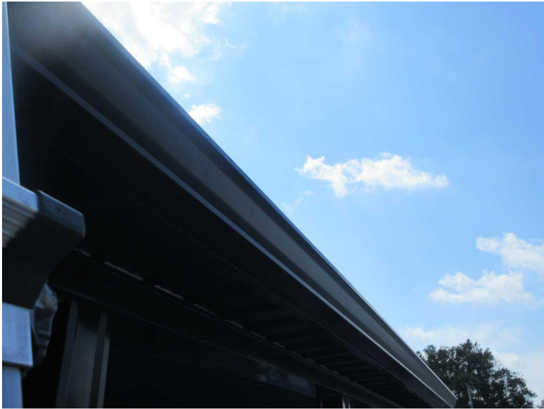
178-Gutters Date Taken: 6/27/2025 Taken By: Michael Wallen Hail damage to gutters.
