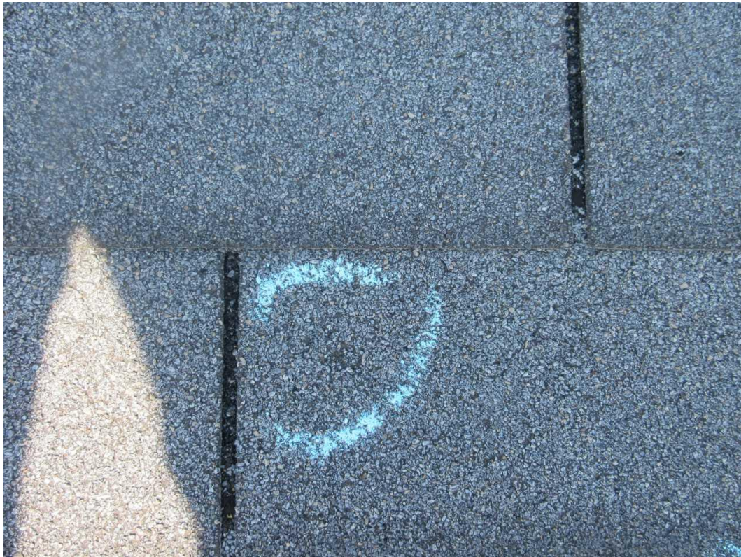
15-E Front Slope Date Taken: 6/27/2025 Taken By: Michael Wallen Close up of hail damage inside the test square.
