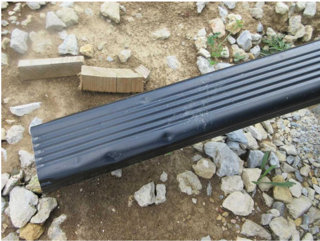
200-N Left Elevation Date Taken: 6/27/2025 Taken By: Michael Wallen Mechanical damage to downspout on the NE corner.
