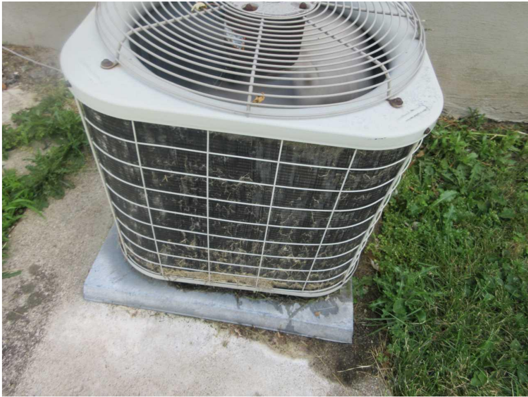
108-W Right Elevation Date Taken: 6/27/2025 Taken By: Michael Wallen Hail damage to A/C fins.
