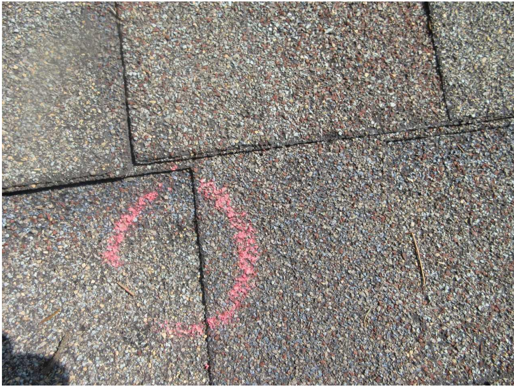
96-S Left Slope Date Taken: 6/27/2025 Taken By: Michael Wallen Close up of hail damage inside the test square.
