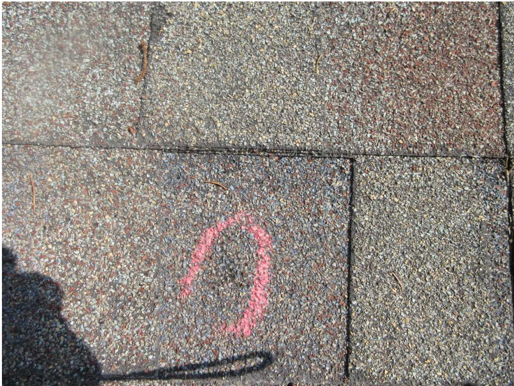
95-S Left Slope Date Taken: 6/27/2025 Taken By: Michael Wallen Close up of hail damage inside the test square.
