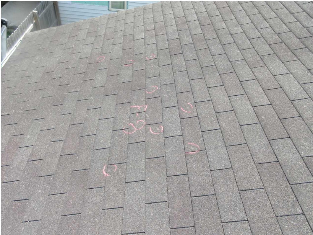
134-N Front Slope Date Taken: 6/27/2025 Taken By: Michael Wallen Overview of the test square.
