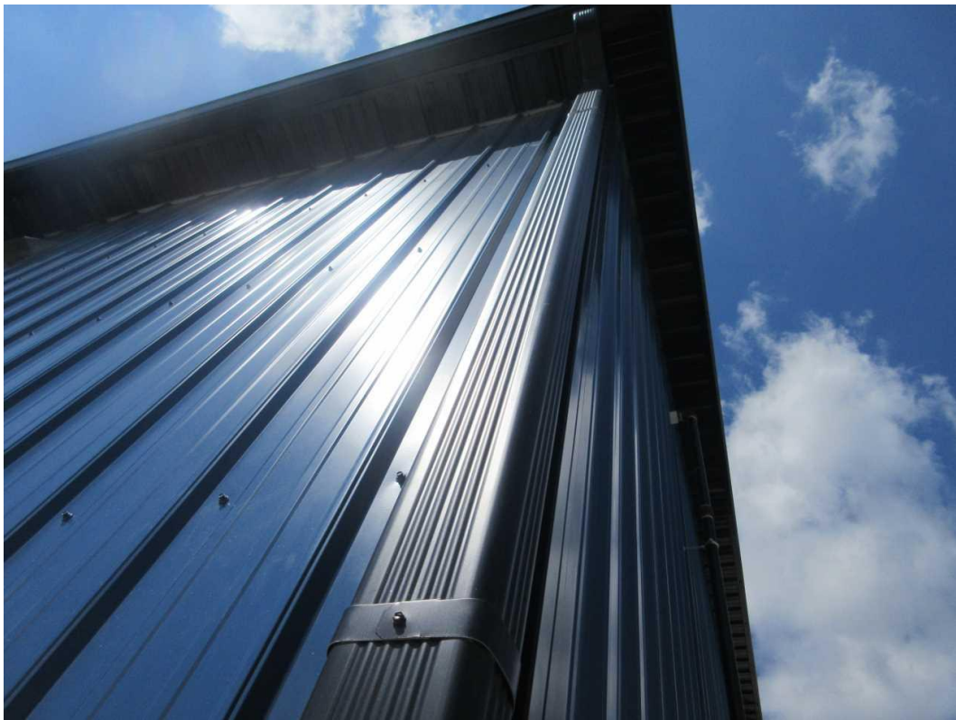
171-E Rear Elevation Date Taken: 6/27/2025 Taken By: Michael Wallen No storm damage to downspout from the claimed date of loss.
