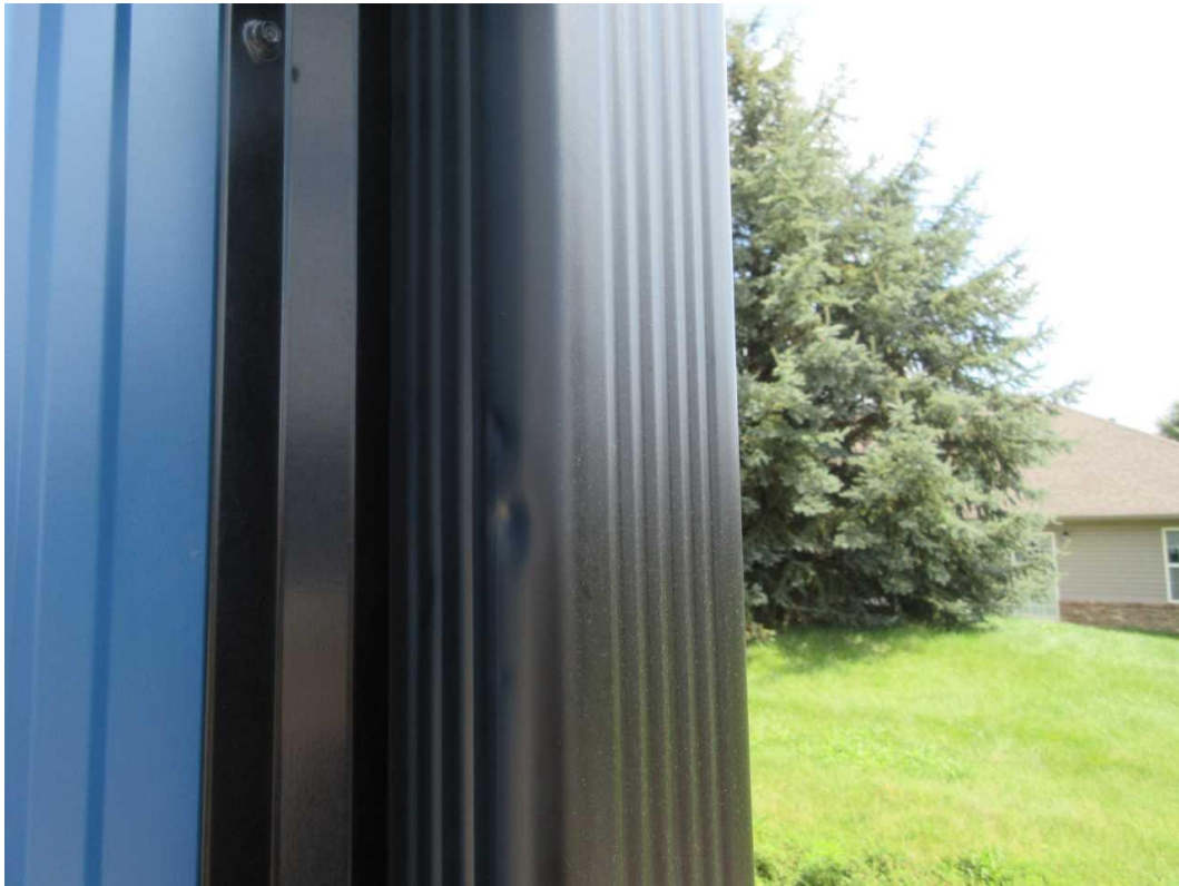
197-S Right Elevation Date Taken: 6/27/2025 Taken By: Michael Wallen Hail damage to downspout.
